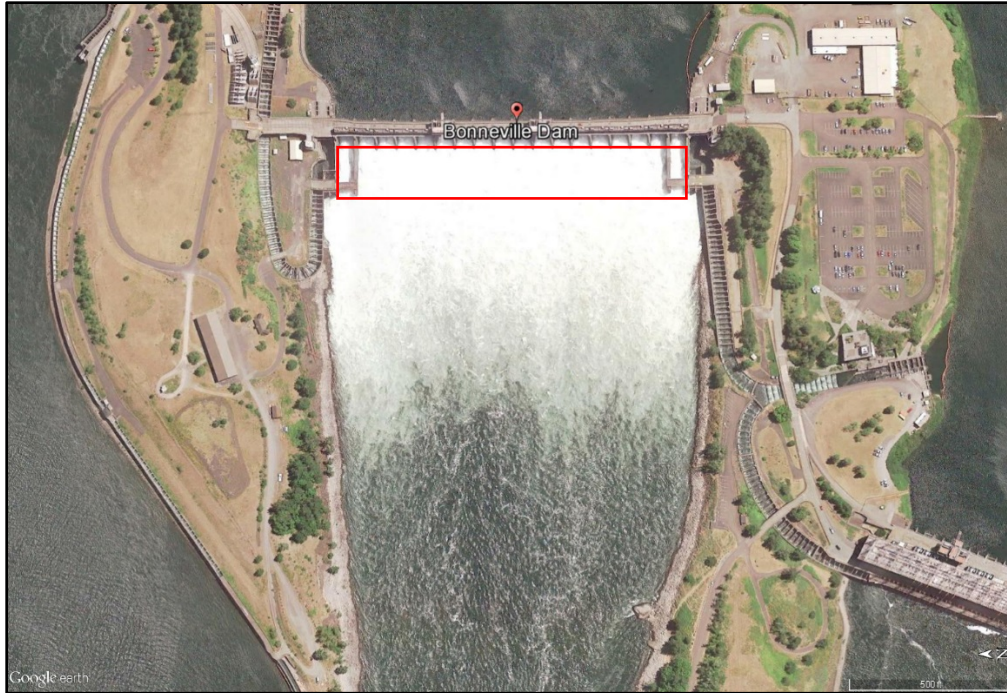
Figure 2 BON Spillway. Red box indicates approximate area of inspection coverage.
