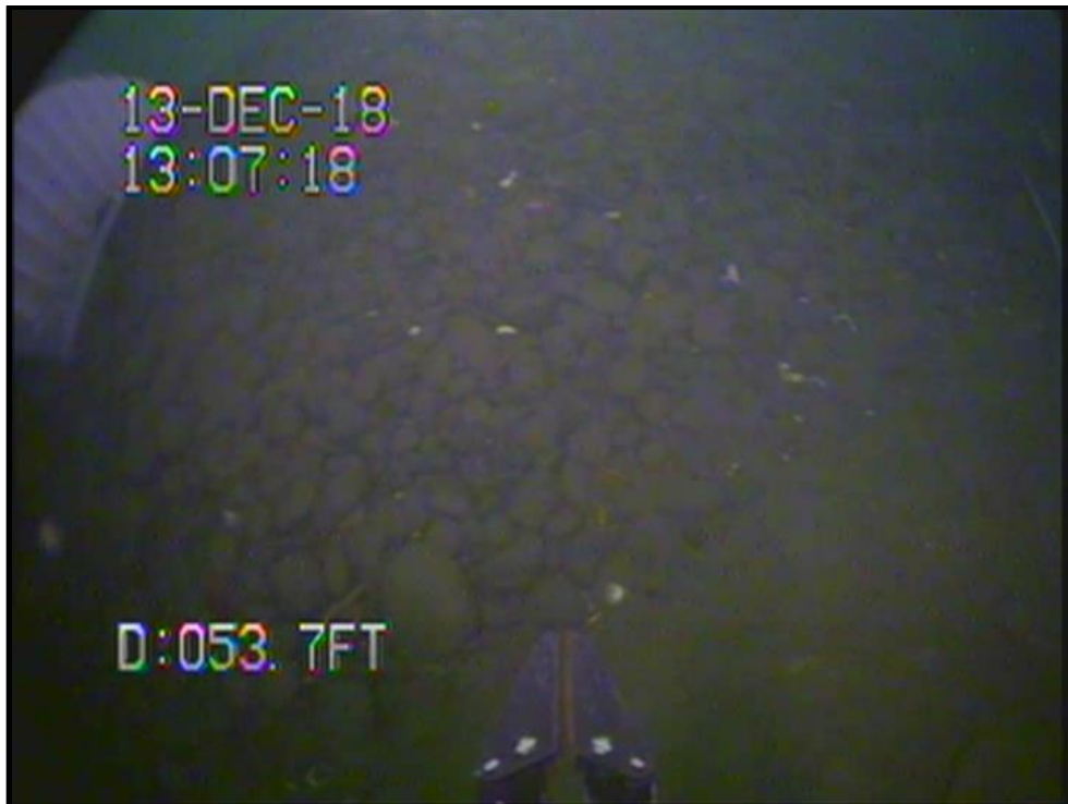
Figure 9 Additional rock at SB 2 End Sill.
