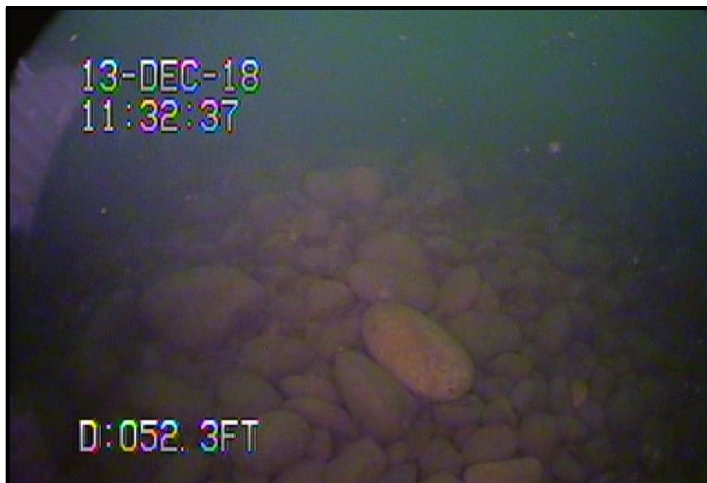
Figure 5 Rock at SB 17 End Sill.
